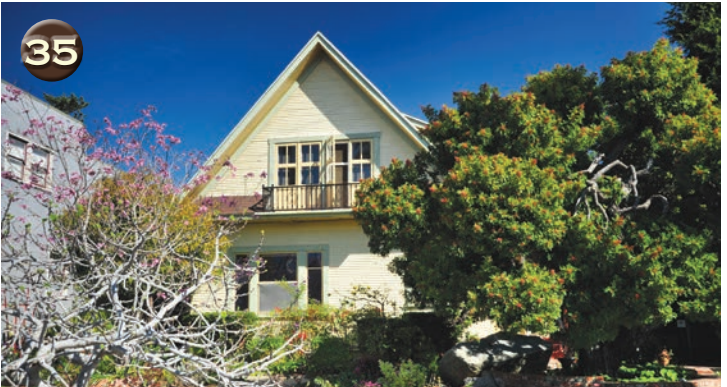
3155 2ND AVENUE CHARLES H. ANTHONY HOUSE, c. 1905 UNKNOWN ARCHITECT COLONIAL REVIVAL
