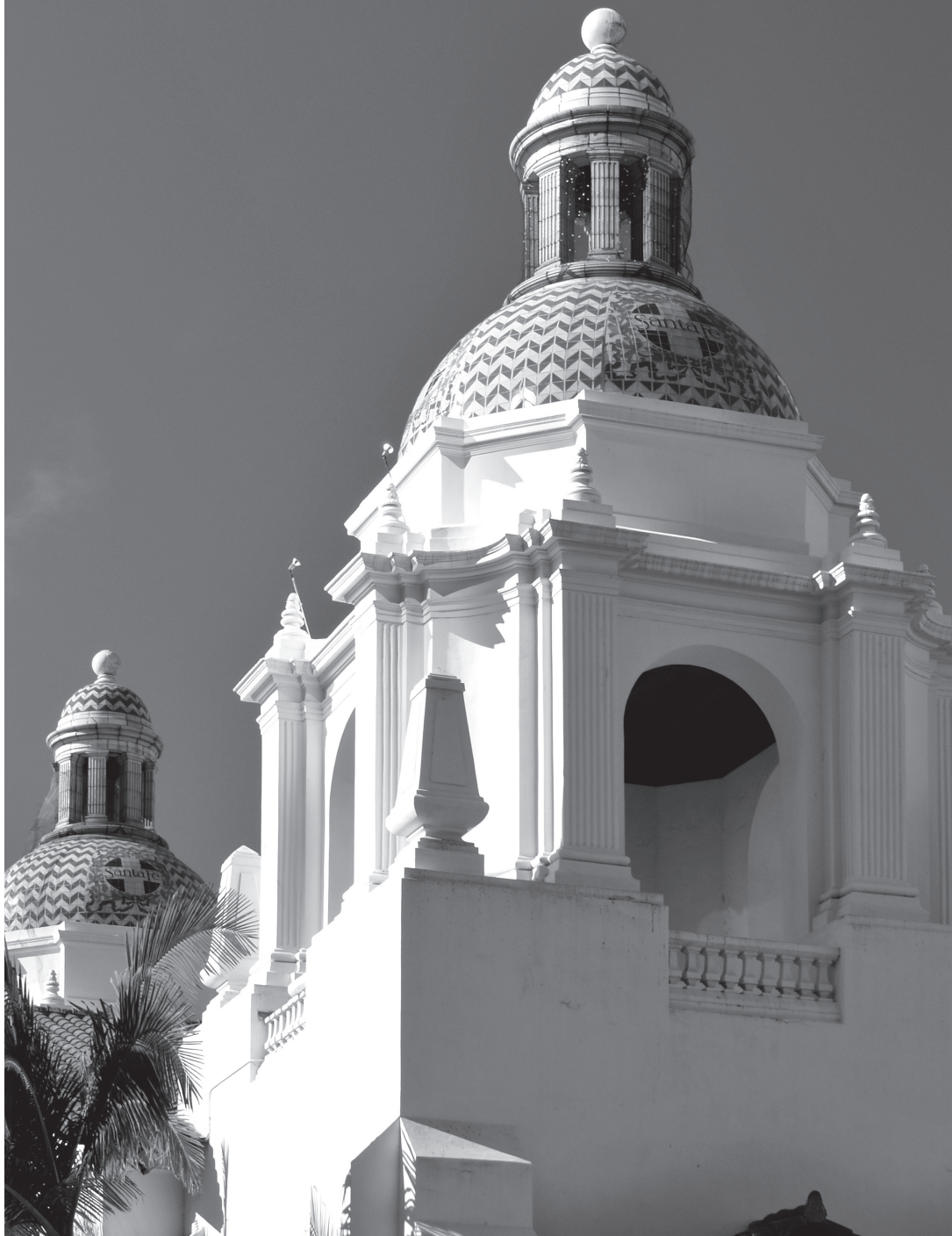
Facing page top California Building; bottom part of an interior wall at the Santa Fe Depot; above tiled domes of the Santa Fe Depot
